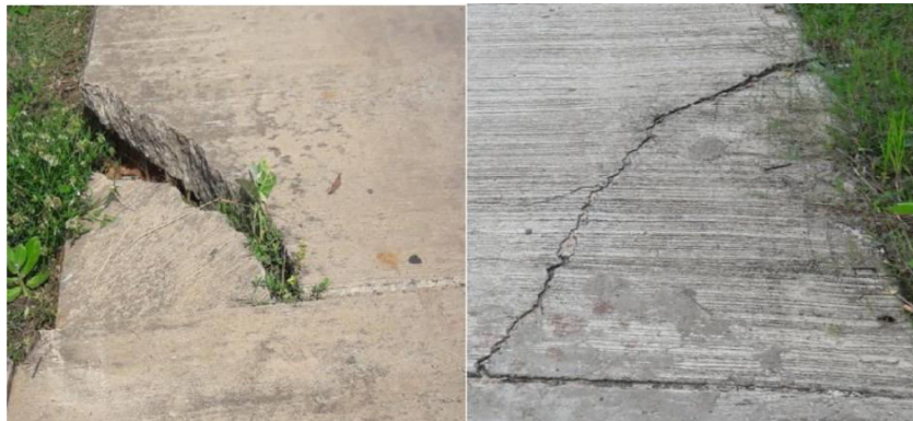
Figure 5. Corner Breaks
