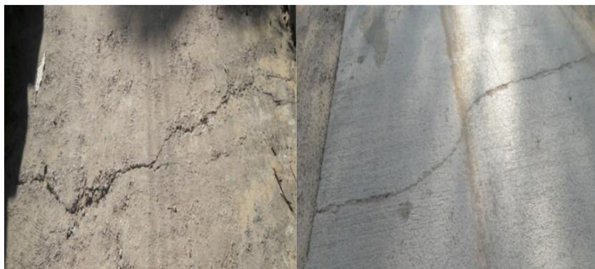
Figure4. Transverse Cracking
